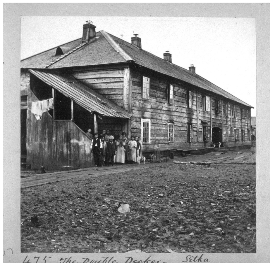
The Double Decker by Eadweard Muybridge, 1868. Over 100 people were listed as living in this building in the 1870 census. Bancroft Library Lone Mountain College Collection
